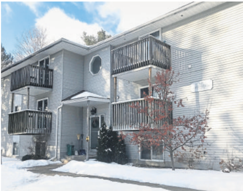
The exterior of building two at 129 Alice Road in Bracebridge.
