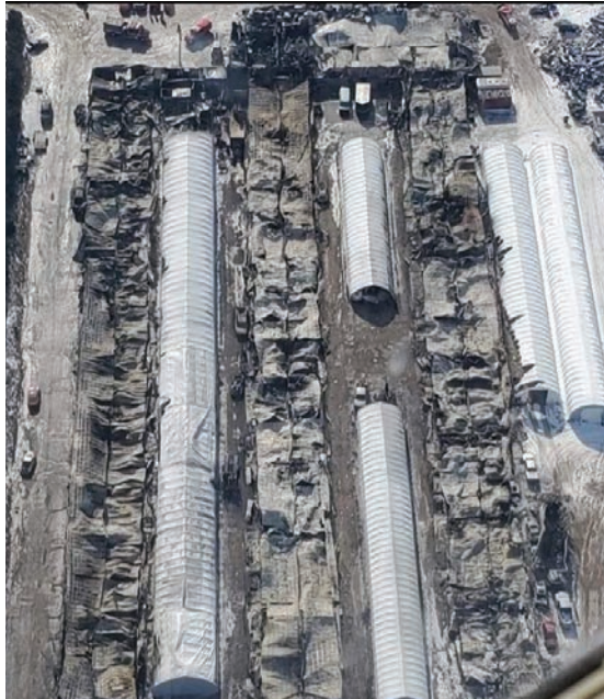
A photo from a GoFundMe for fire victims shows an aerial view of the destruction. SOURCED
