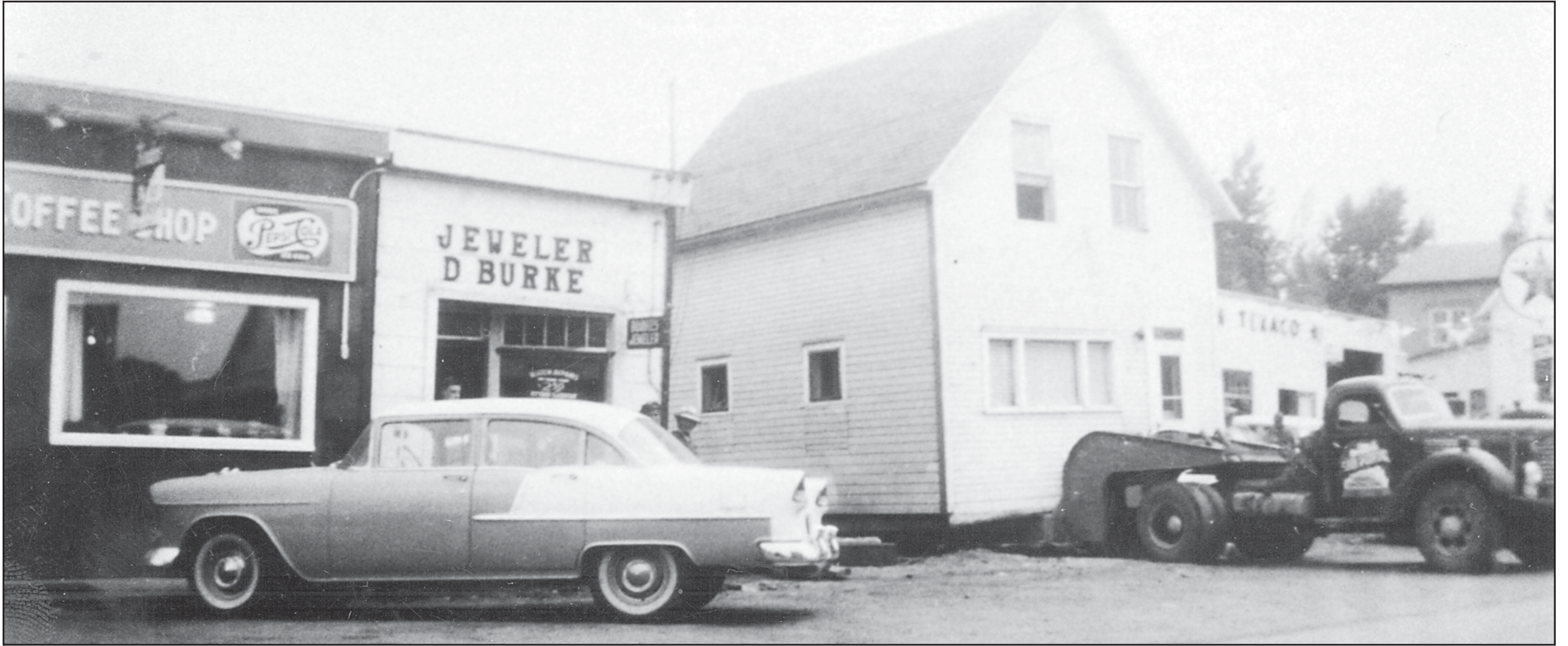
Queen Street in Killaloe was a busy place with a store, coffee shop, jewelry shop, car dealerships, garages and more. In this photo, the white building in the photograph is being moved and is now located near the curling club. At the far right of the picture, Calvary Baptist Church can still be seen on the hill, probably the only thing in the photo which has a semblance still today. (Photos courtesy Pearl Murack.)
