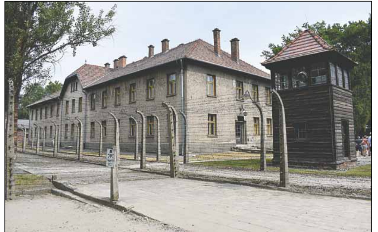
The commandant's and administration building, Auschwitz I.
