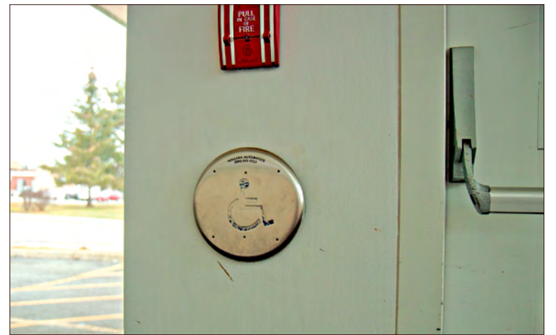
A handicapped access button inside the front entrance. VOICE PHOTO
