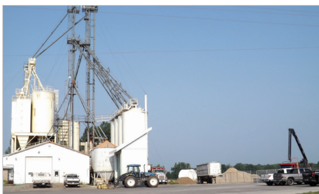
Seed facility - Construction of a state-of-the art seed processing, treatment and packaging facility at the Snobelen Farms Ltd. Palmerston area location will get underway this summer, the company announced last week. Photo by Patrick Raftis
